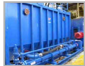
High Pressure hydro-cyclone feed for mud cleansing
