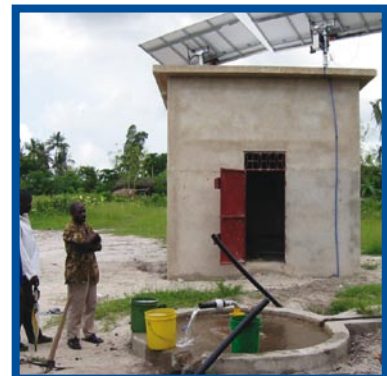
Commissioning the new water supply.
