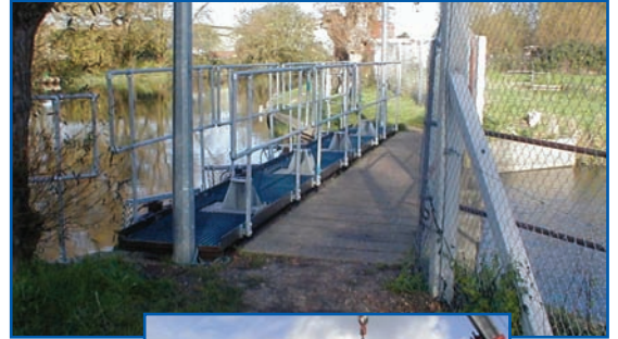
A walkway installed as part of a river intake contract
