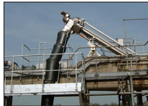
Screw Conveyor installation at a local treatment works
