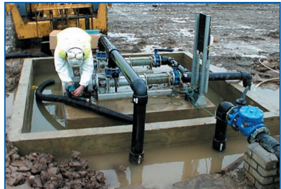
Duty/standby pump installation
