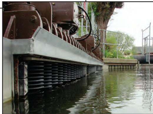
4 Discreens installed at a lagoon intake to screen abstracted water
