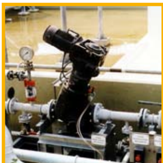
A Muncher macerating solids in secondary liquid fuel to prevent blocking pumps and filters
