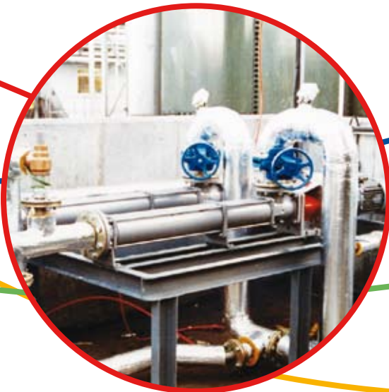
Pumping of slurry mix
