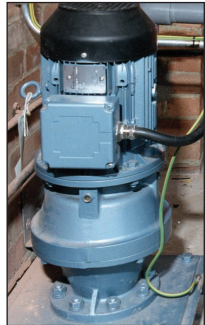
M180 mm Vertical Macerator installed as part of a pumping system to handle sewage from a primary school.
