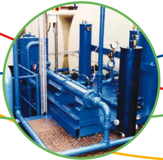
Transfer of hydraulic/ waste oil
