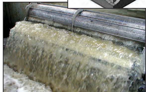
2 Stormscreens installed to screen storm overflows
